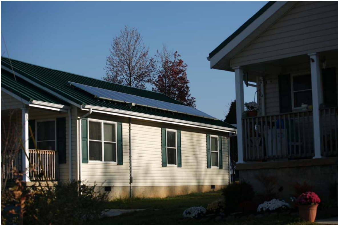
Figure 45. Solar modules sit very nicely on the roof of ZEH2. The dark green roof makes for a very pleasing appearance with the dark bluish-green polycrystalline module
