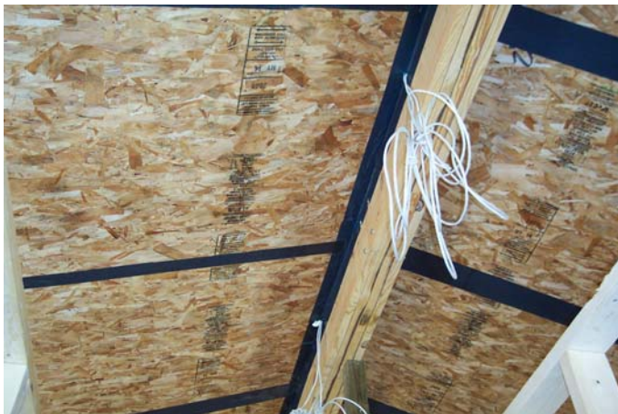
Figure 40 Wires being pulled into the space above the ridge beam.
