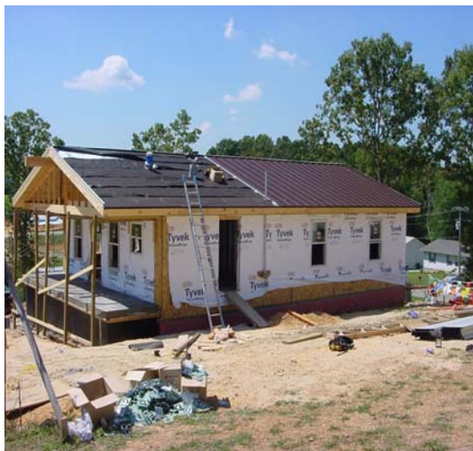
Figure 29. Roof drainage plane under the raised metal roof.
