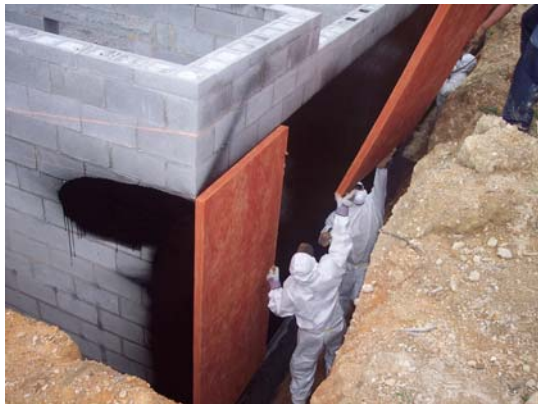
Figure 22. Installation of four by eight foot fiberglass boards sized to cover the waterproofing
