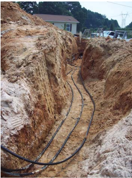
Figure 34. Geothermal pipe being installed in the sewer trench.
