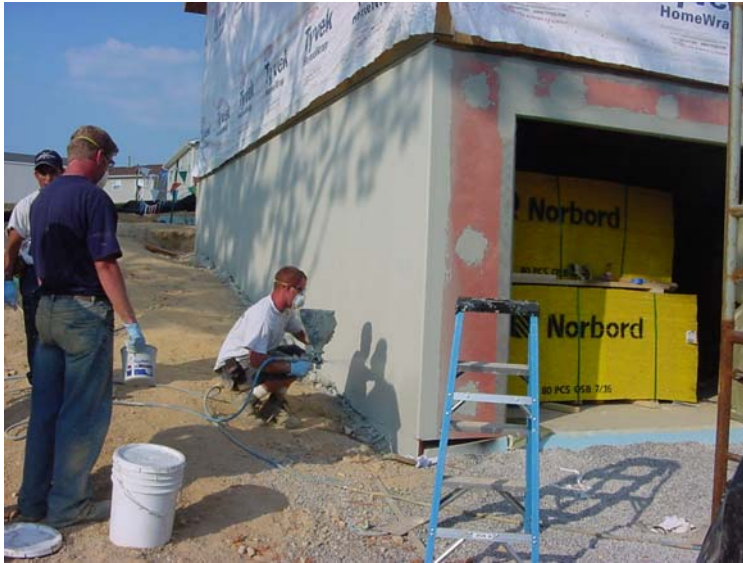
Figure 24. The above grade portion of the foundation wall receiving final spray covering.
