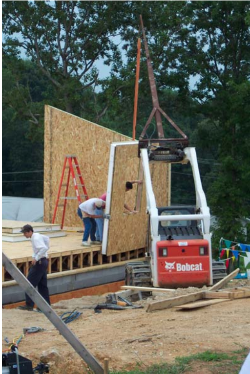
Figure 42. Mounting the wall panels on the side of the floor trusses leaves easy access to run electric wires from the basement into the vertical wiring chases in the wall SIPs.
