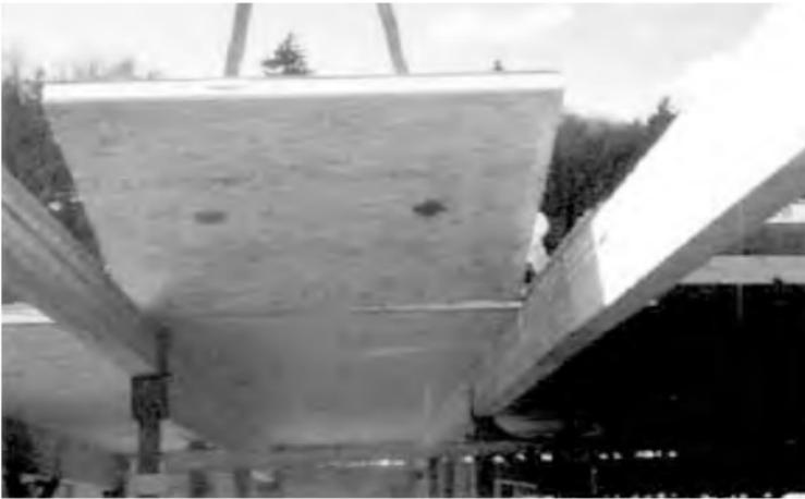
Upon receiving your roof panels, count them and check the sizes. In most cases roof panels are not fabricated at the factory because roofs tend to vary from the shop drawings. If they have been factory fabricated, double check for accuracy. Also, check the edge treatment. You may have to plane your lumber or I-joists to fit the recesses. If the panels aren't being installed immediately, cover the panels and lumber until ready for installation.
