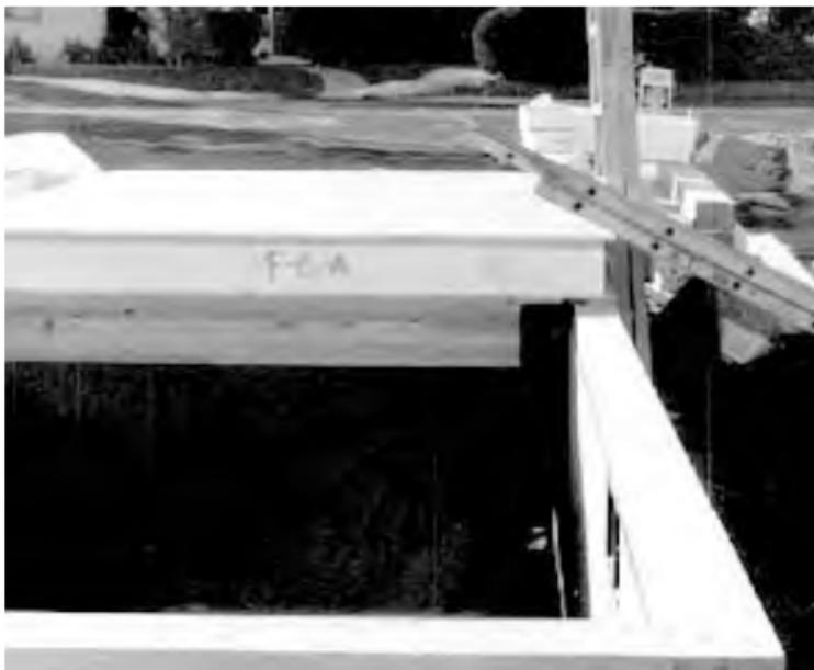
Use only one nail into each 4' spline to hold it in place. Do not nail off the spline until the next panel is in place. Refer back to the connections section for proper mastic placement.
