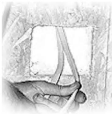
Use vertical chases and interior walls whenever possible for most of your wiring needs.
