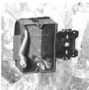
Where walls terminate against a panel you can drill (at the horizontal electrical chase height) a long diagonal hole through the face of the stud diagonally into the electrical chase. Electrical wires will stuff easily into this type of access.
